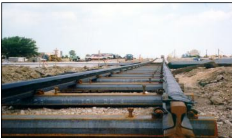
Embedded track construction with new continuous welded rail wrapped in the Ironhorse “Boot”®, fastened to steel ties.
