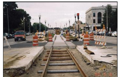
By using steel ties where track runs through pavement, the cost of the in-street track was reduced.
